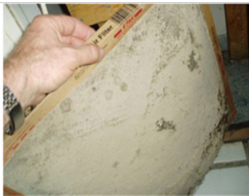
How's the filter? A clogged low efficiency filter partially sucked out of the frame.
