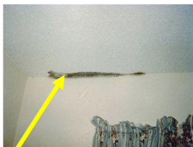
Mold due to poor insulation or wind blowing through insulation.
