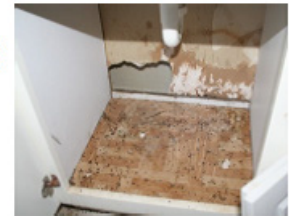
Roach frass under sink
