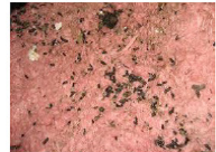
Rat feces in insulation
