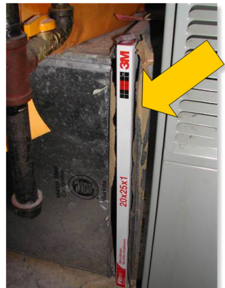
Poorly sealed filter access panel
