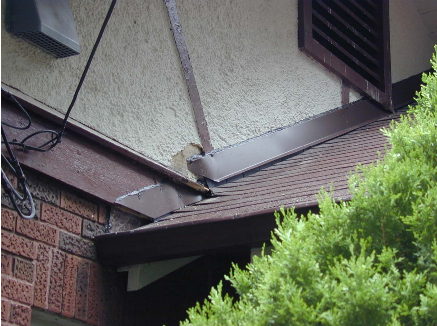
Exercise 5: Identify the Moisture Problems
