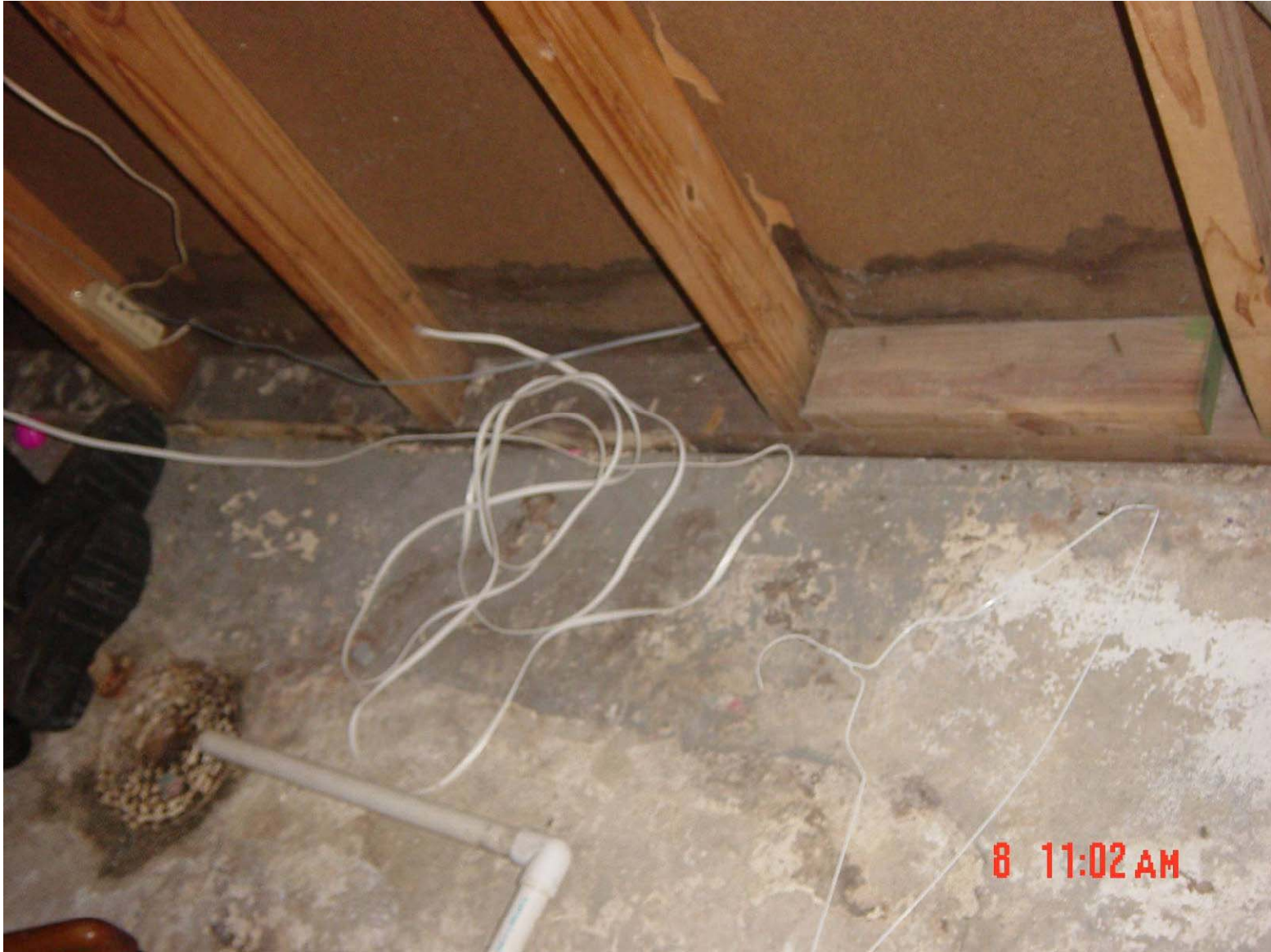
Exercise 5: Identify the Moisture Problems
