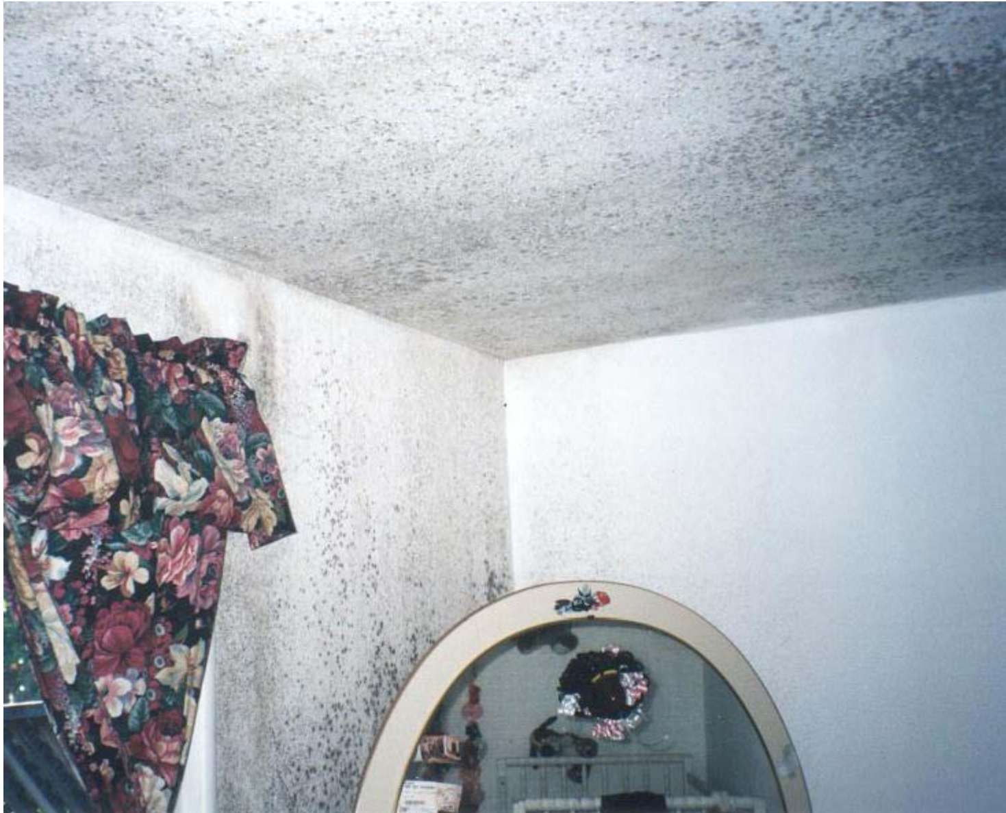
Exercise 5: Identify the Moisture Problems
