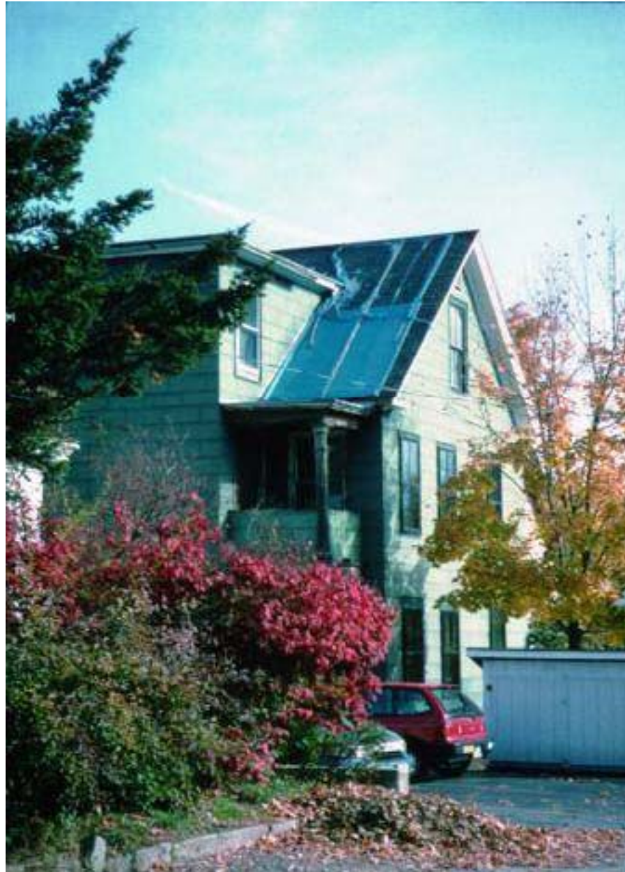
Exercise 5: Identify the Moisture Problems
