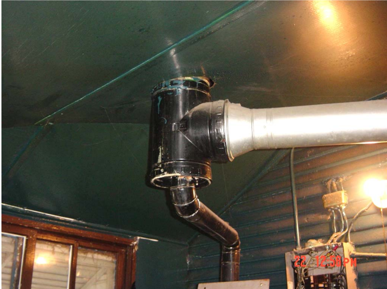
Exercise 7: Identify the Ventilation Problems
