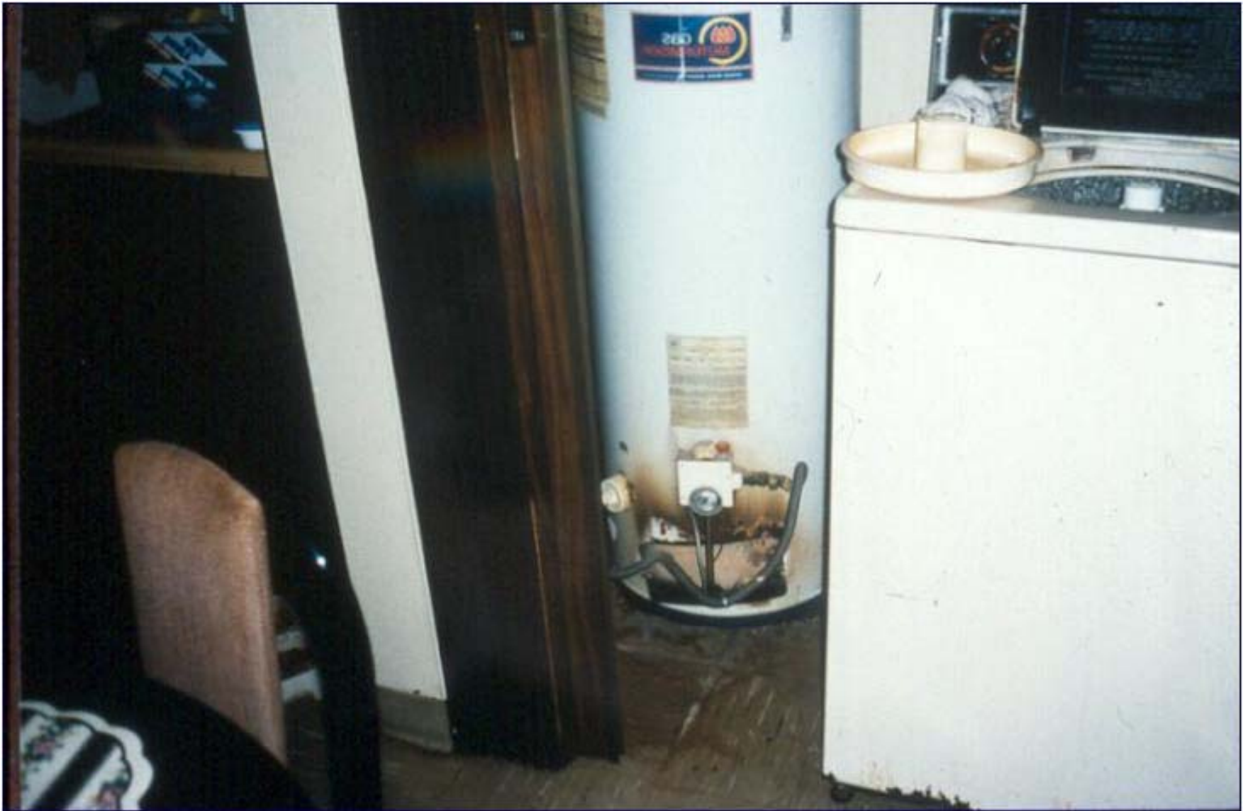
Exercise 7: Identify the Ventilation Problems
