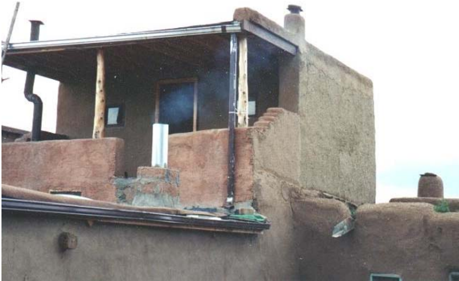
Exercise 7: Identify the Ventilation Problems
