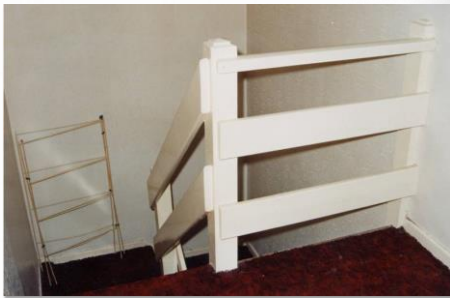
Falling on stairs and falling between levels
