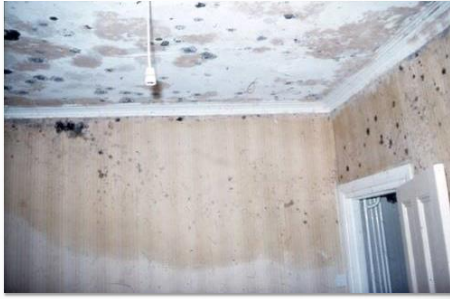
Mold and moisture
