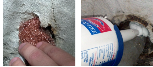
Fill larger gaps with copper mesh (left). Seal gaps around pipes with caulk (right). Photos: Mary Maley, Northeastern IPM Center.
