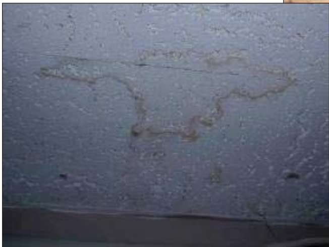
Rodent urine stain in drop ceiling
