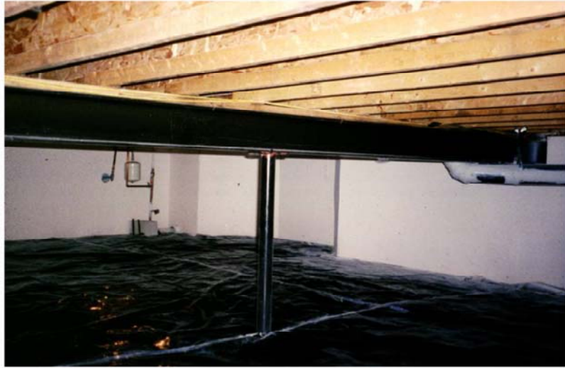
Good Sealed Crawlspace
