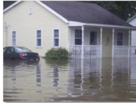
Moisture/ water intrusion
